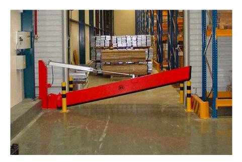
Automatic closing activated by signal from your fire detection or leak detection system or by push button. Push button to open / reset.
